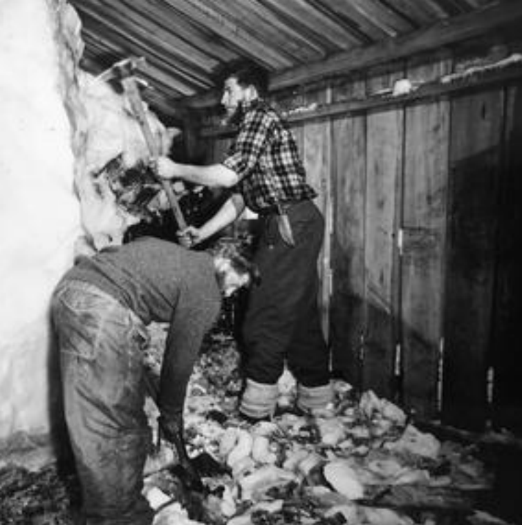
Bob Buckley (top) and Colin Jenness clearing ice in the wooden annexe to the Cape Evans Hut. Lack of time prevented further progress in this area and followed the removal of approximately 200m 3 from the main building. Quartermain said, “Bob Buckley is an absolute bullock for work—at least in spasms—and when he yields a pick the hard ice just crumples up.’
