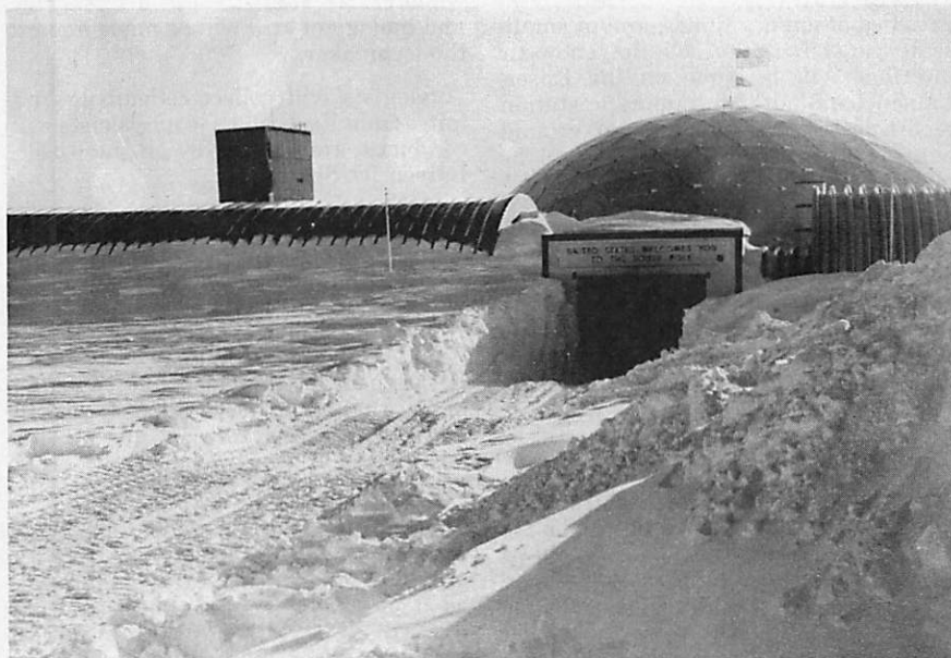
Winter snow in high drifts at the entrance to the geodesic dome complex at the Amundsen-Scott South Pole Station. When daylight and fine weather returned the 18 men who wintered at the Pole this year had a lot of snow clearing to do.
