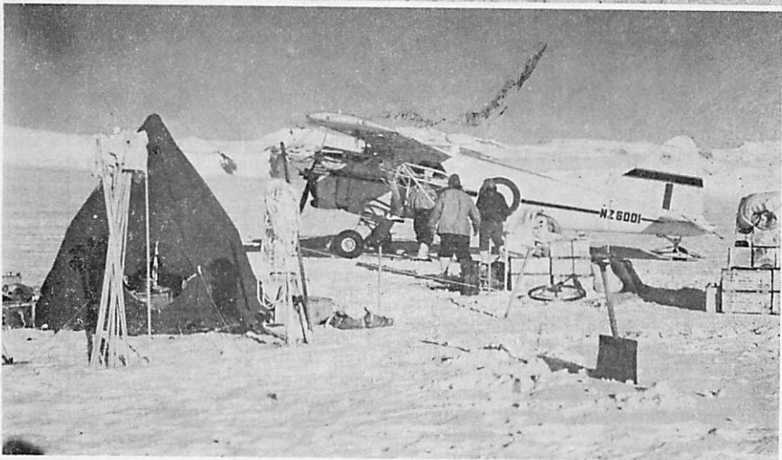
FIRST ARRIVALS —Above: Scott Base under construction in January, 1957. At the right is a Ferguson tractor in its original state before modification for the Pole journey. Below: A Beaver aircraft of the Royal New Zealand Air Force Flight at the Skelton Glacier depot camp in the first year.
