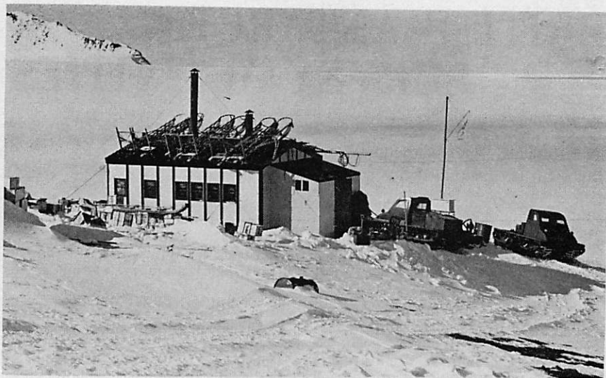
This small building with vehicles at the front door and sledges on the roof is the British Antarctic Survey advance base at Fossil Bluff. It stands on Alexander Island above George VI Sound, Antarctic Peninsula.
