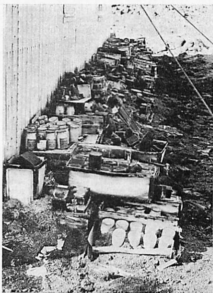
Sixty-year-old stores stacked against the outside wall of the Shackleton Hut.
